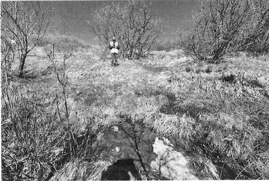
Left abutment seepage area
