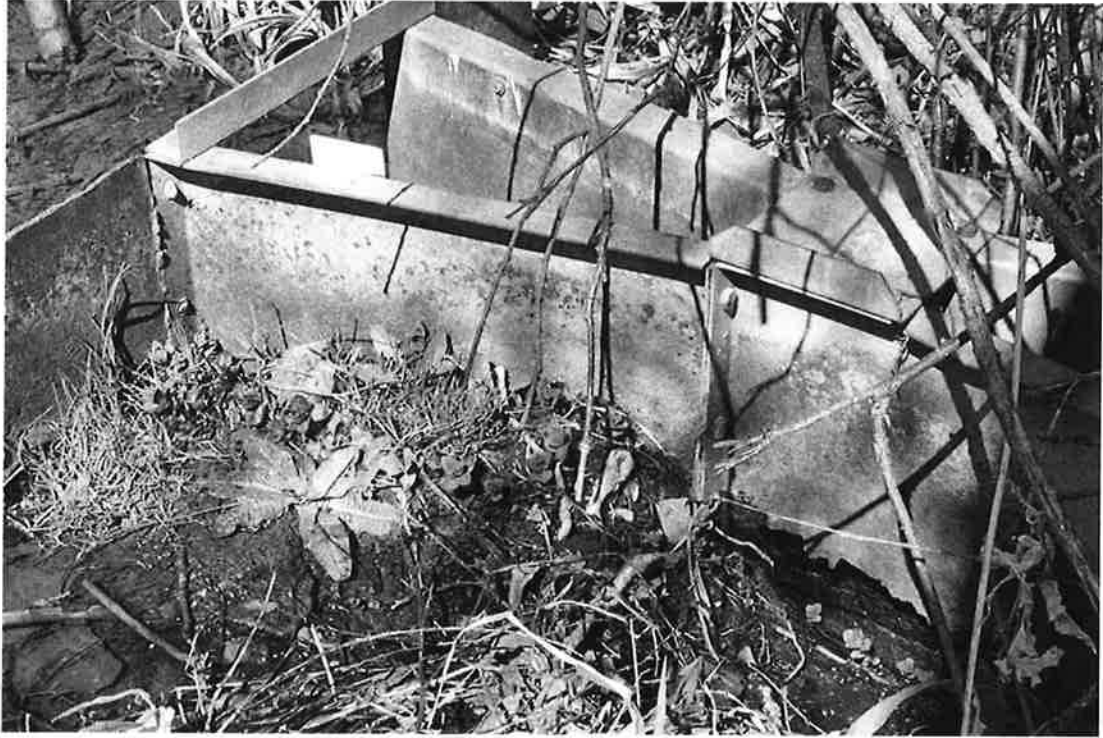
Corroded Parshall flume (subsequently repaired)
