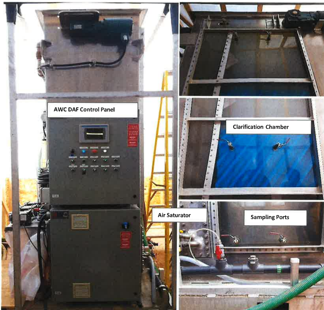
Image 1: AWC Pilot DAF Skid System – Control Panel and Clarification Column
