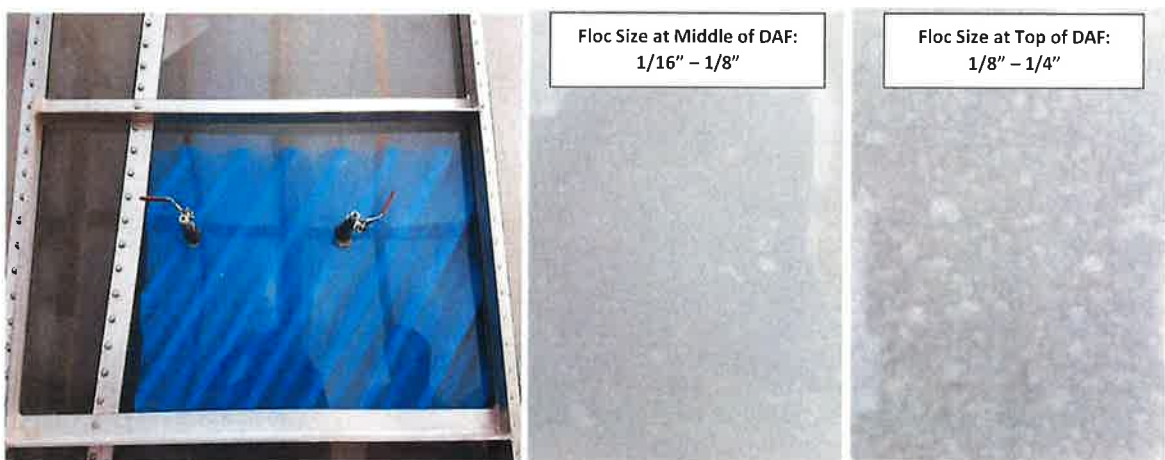
Image 4: Saturated Air Mixing Zone (Clarification Chamber) – Formation of Floc, Baffles, and Approximate Floc Sizes
