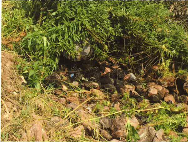
Figure 4 – CCMD WWTP Effluent Outfall
